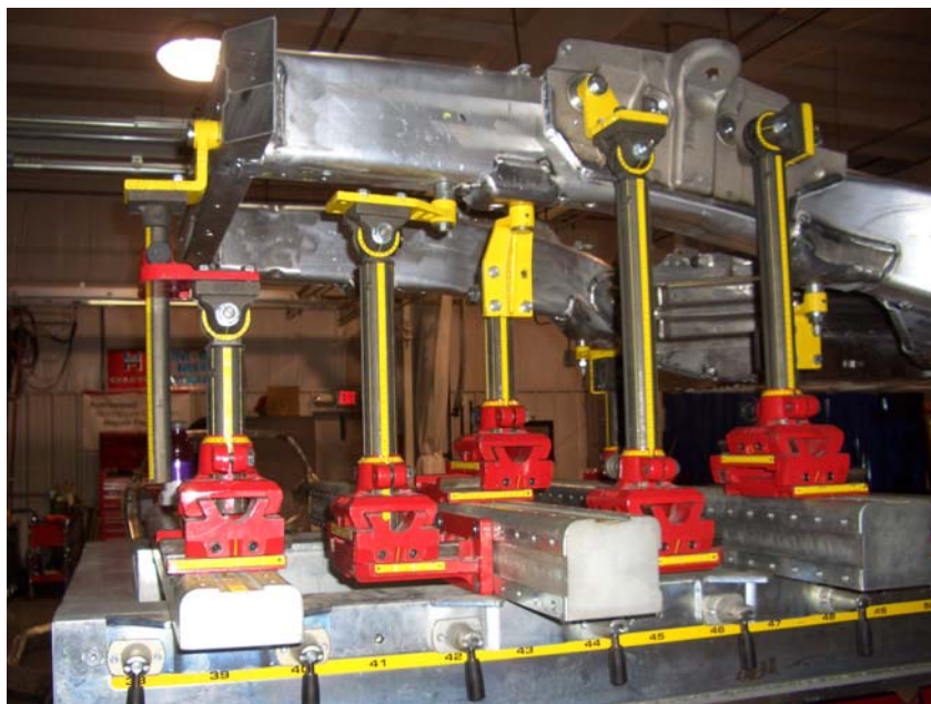
The new rail is bolted to the jigs and welded in place.
